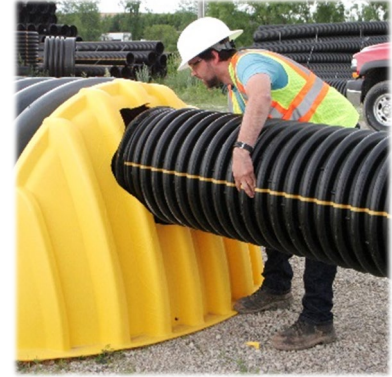
Figure 4: Inserting the Pipe
