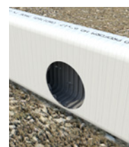
Cut using a 4" hole saw
