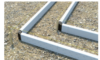
Spacer straps and string lines
