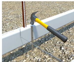
Tap pin to desired elevation
