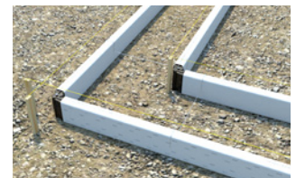
Spacer straps and string lines
