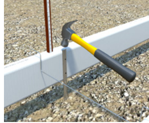
Tap pin to desired elevation
