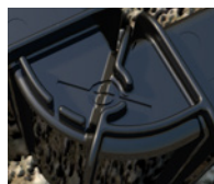
Location for rebar
