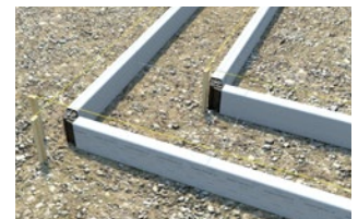
Spacer straps and string lines
