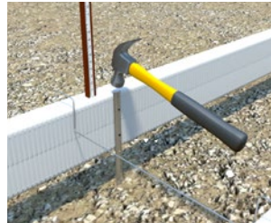
Tap pin to desired elevation
