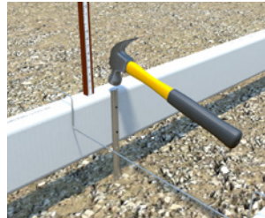
Tap pin to desired elevation
