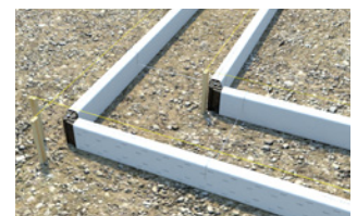
Spacer straps and string lines
