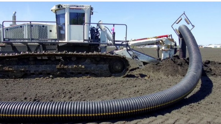
Goldflex flexible dual-wall feeds directly from a stringer to a plow boot
