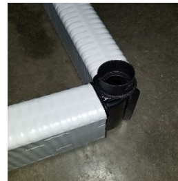
Figure 4: Installed port on PFHD 90° Elbow
