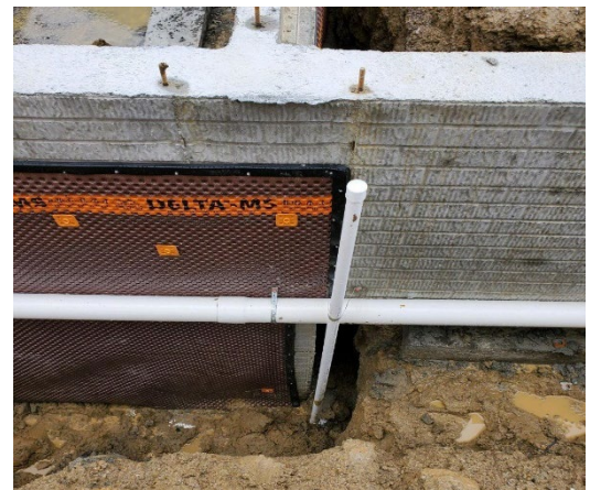
Figure 7: Installed Inspection Port with PVC pipe.
