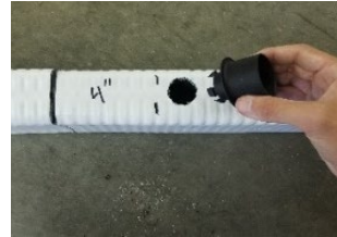
Figure 1: Inserting into PFHD stick.
