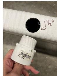
**Figure 1: Inserting into PFHD stick.**
