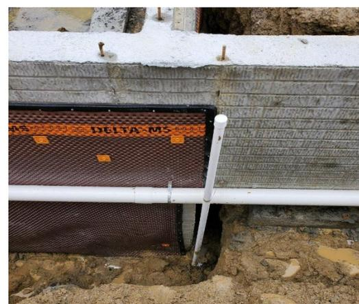
**Figure 7: Installed Inspection Port with PVC pipe.**
