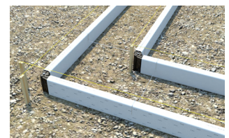
Spacer straps and string lines
