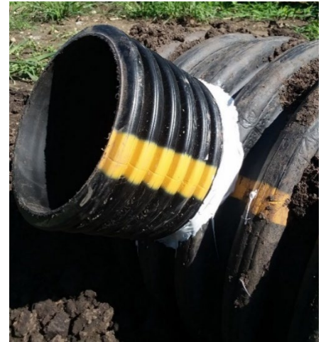
Figure 4: Installed GOLDFLO Tap Tee
