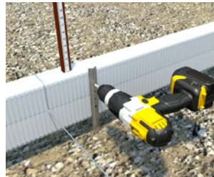
Use short screws or nails to fasten pin
