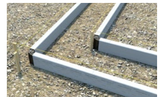
Spacer straps and string lines
